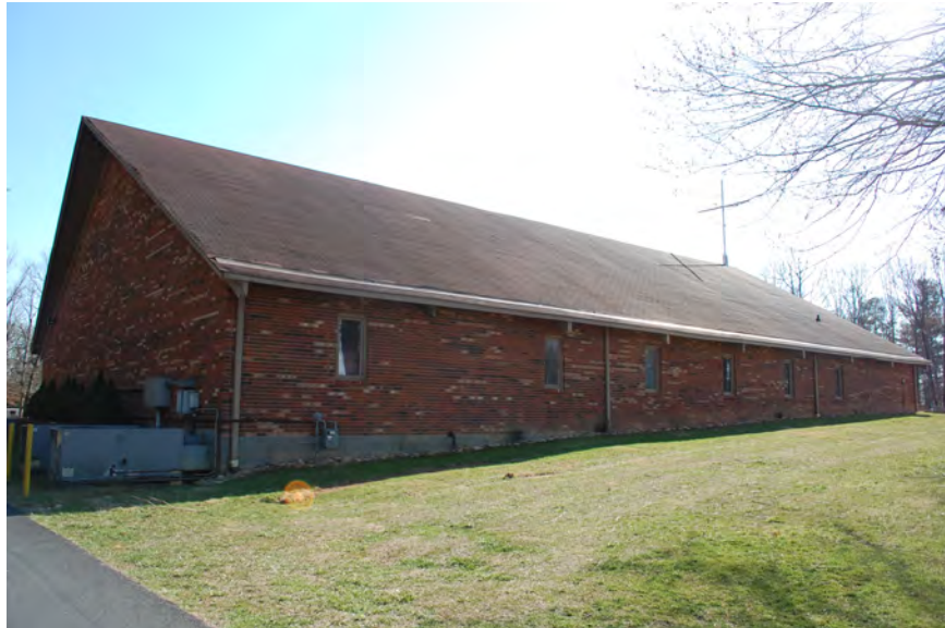
Figure 115: 1979 church, facing southwest
