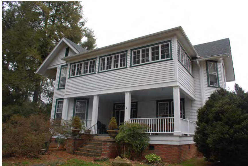
Figure 33: McMurray House, facing northeast
