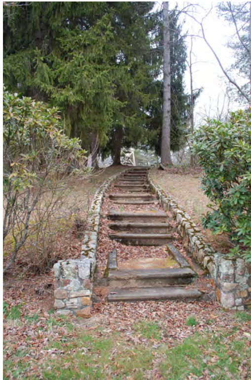
Figure 64: Stairs above campfire area, facing north
