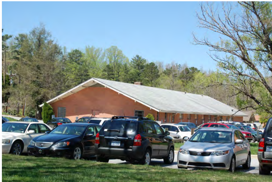
Figure 84: Circa 1970 medical building on southwest corner of the quad, facing northwest
