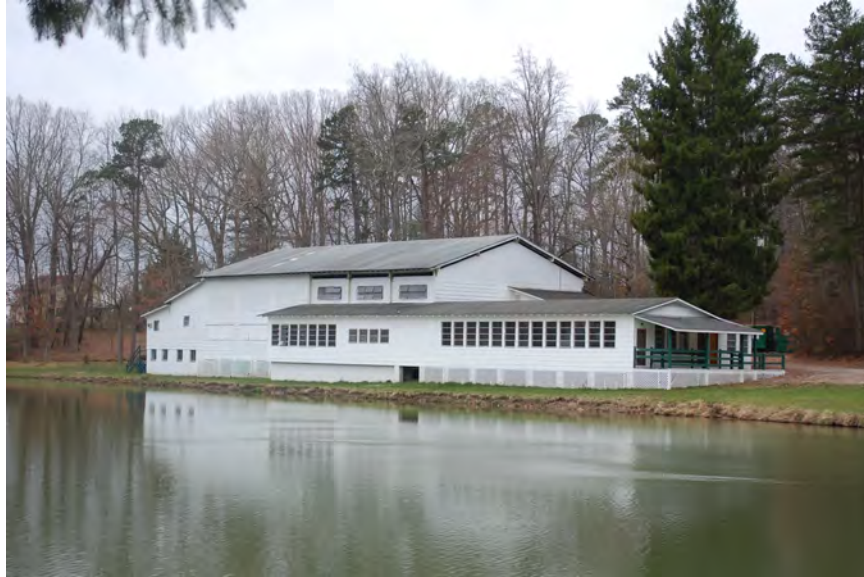
Figure 56: Camp Pinewood Lake and dining hall and gym, facing southwest
