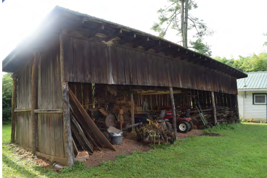
Figure 45: Shed, facing southeast
