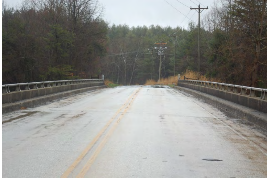
62. Brookside Camp Road Bridge 1963
