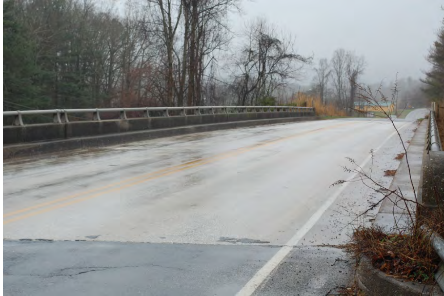
60. Meadowlark Lane Bridge 1964
