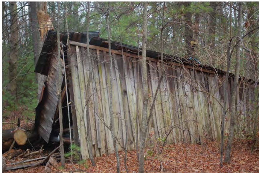
Figure 103: Vertical-board shed, facing west
