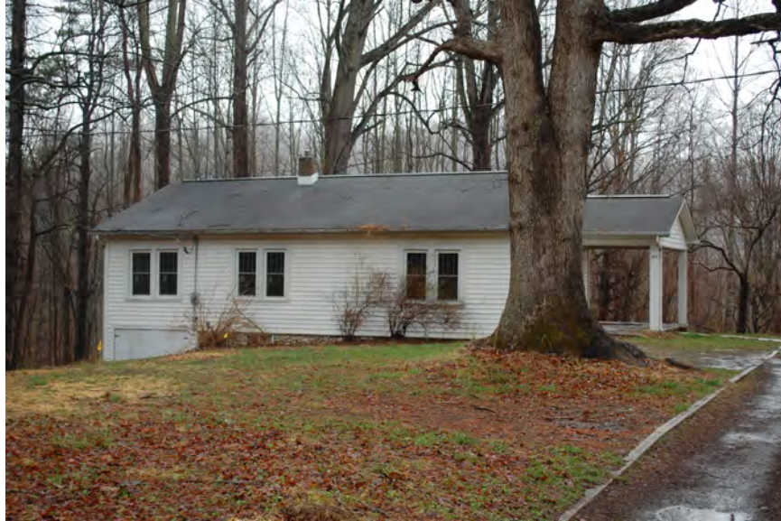
Figure 91: Circa 1930 bungalow on east side of Howard Gap Road, facing east
