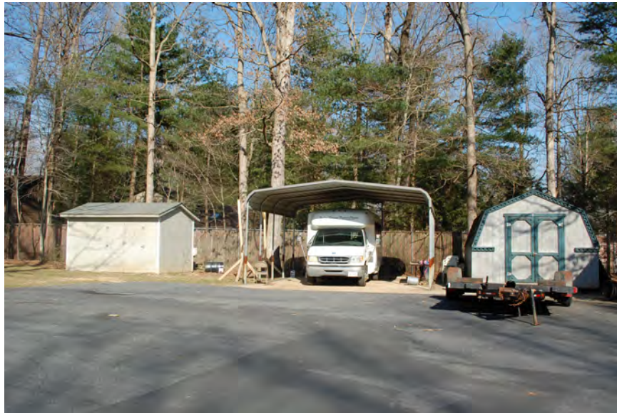
Figure 122: Prefabricated buildings/structures north of fellowship hall, facing east
