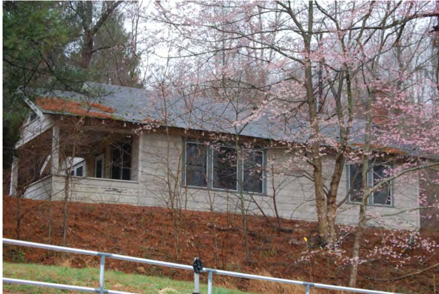
Figure 95: Circa 1930 bungalow on west side of Howard Gap Road, facing southwest
