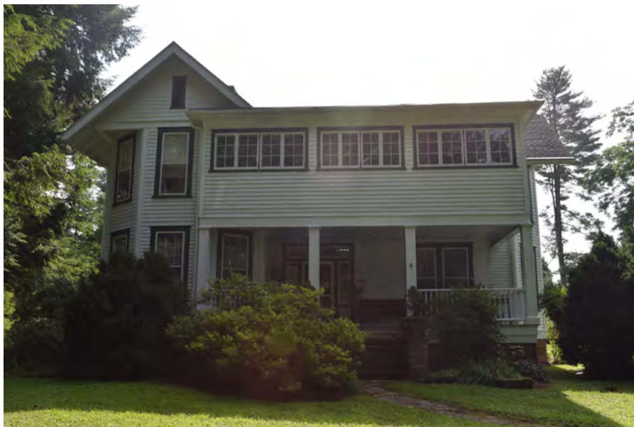
Figure 37: McMurray House facade, facing east
