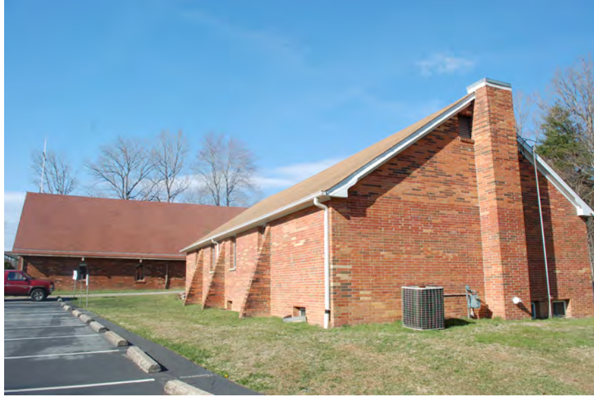
Figure 118: 1964 chapel, facing north-northeast
