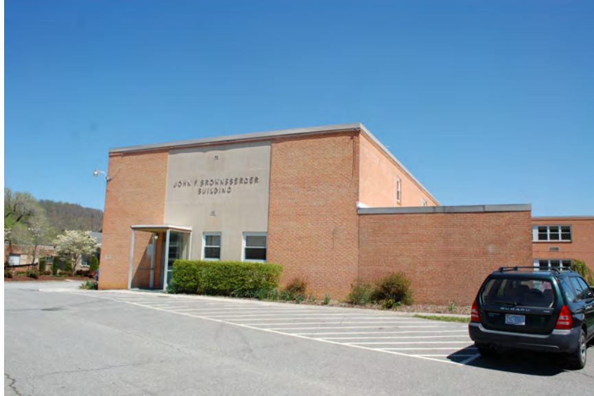
Figure 73: Circa 1950 hospital, facing east-northeast
