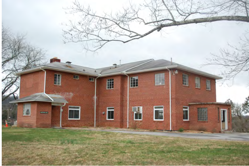
Figure 77: Circa 1960 cafeteria building, facing southeast
