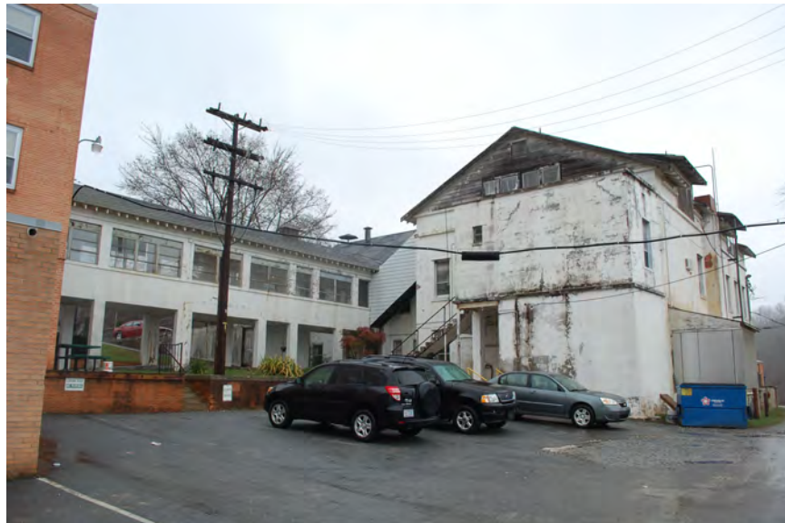
Figure 82: South side circa 1930 hospital, facing north-northwest
