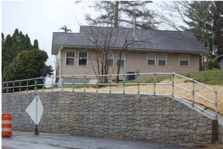
Figure 94: Circa 1940 bungalow on west side of Howard Gap Road, facing southwest
