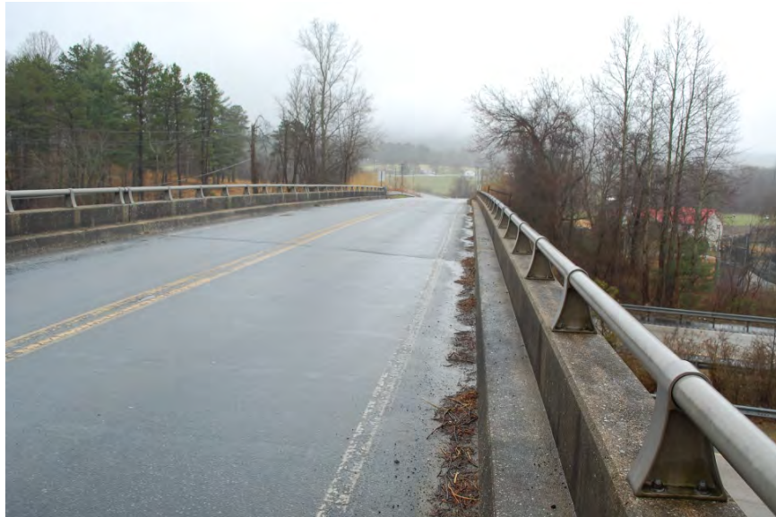
63. Naples Road Bridge 1963
