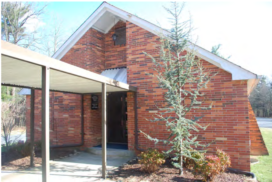
Figure 117: 1964 chapel, facing south-southeast
