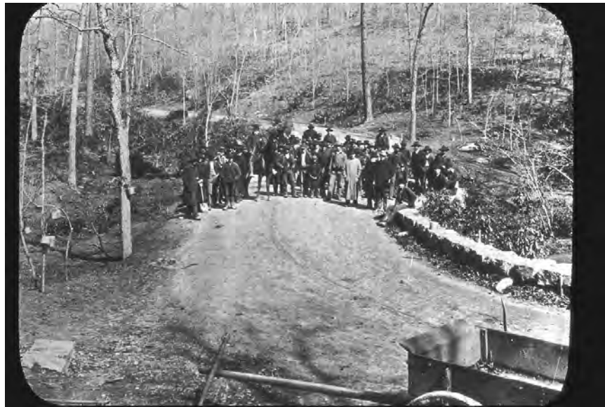
Figure 19: Approach road under construction, circa 1895, from the Library of Congress
