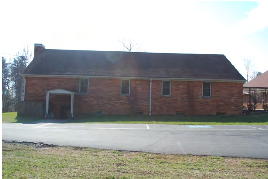
Figure 119: 1964 chapel, facing west
