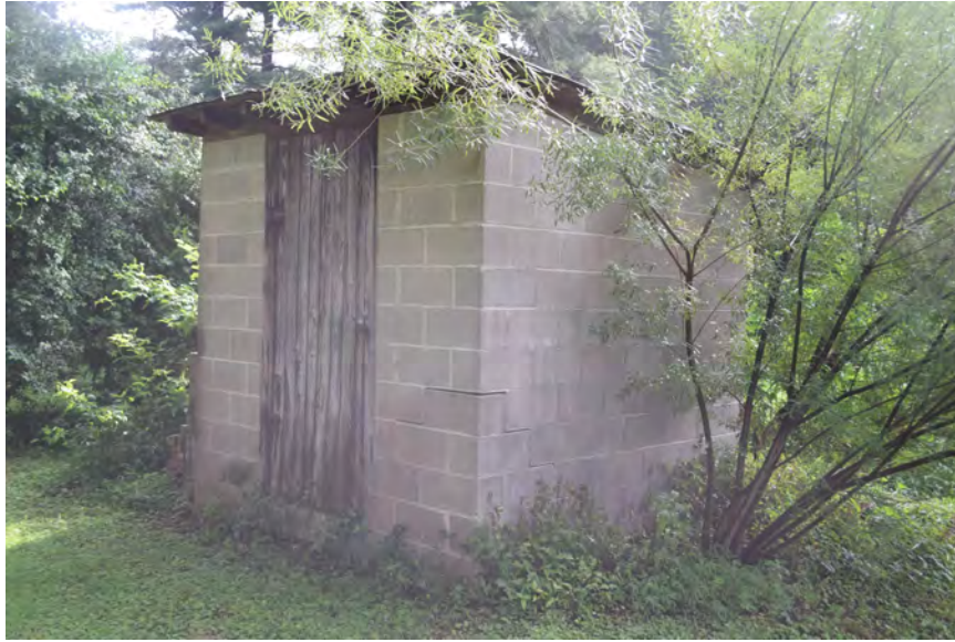
Figure 49: Smokehouse, facing west
