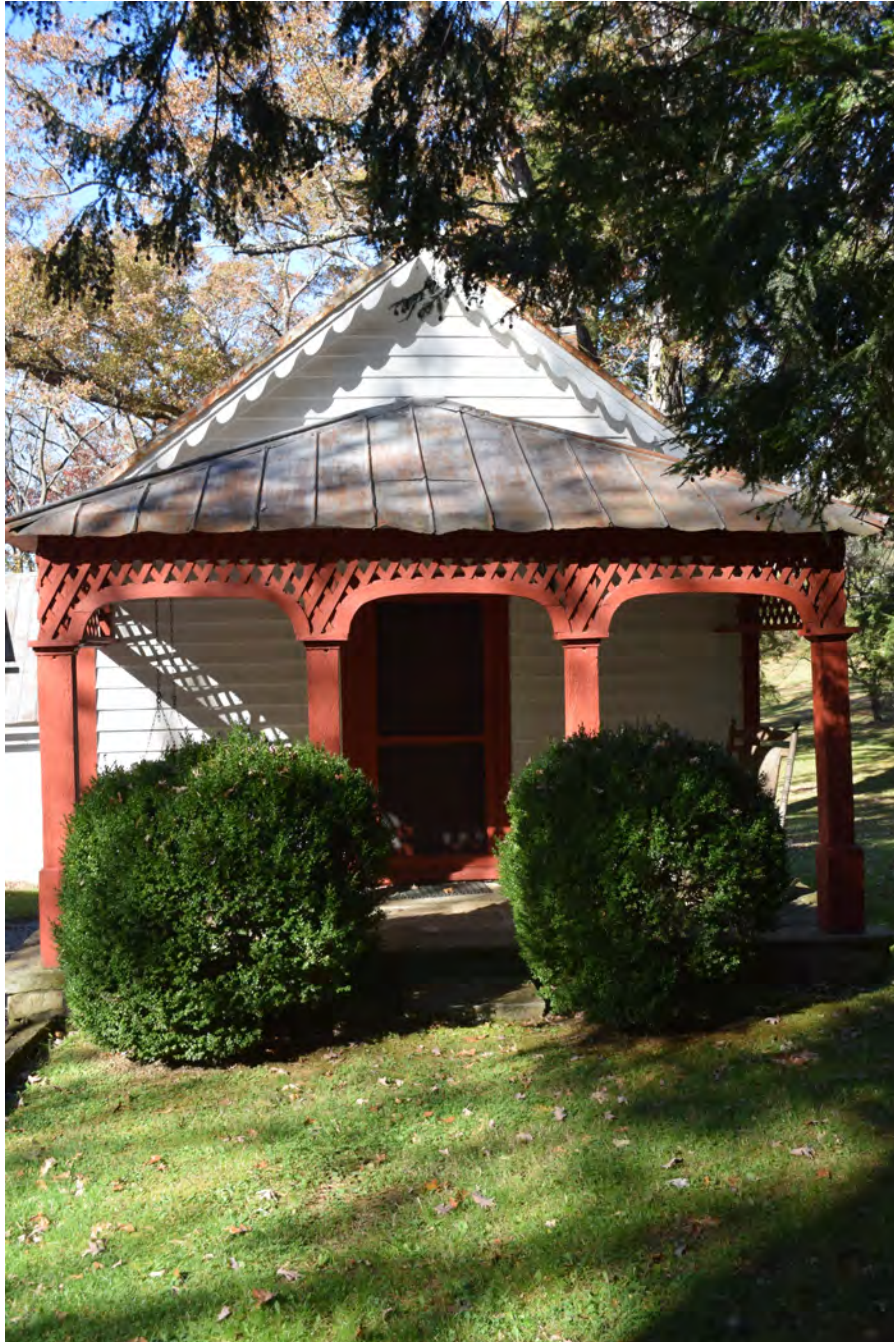
Figure 9: Office/Ice House, facing north-northeast
