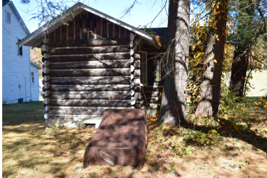
Figure 25: Log Cabin, facing north
