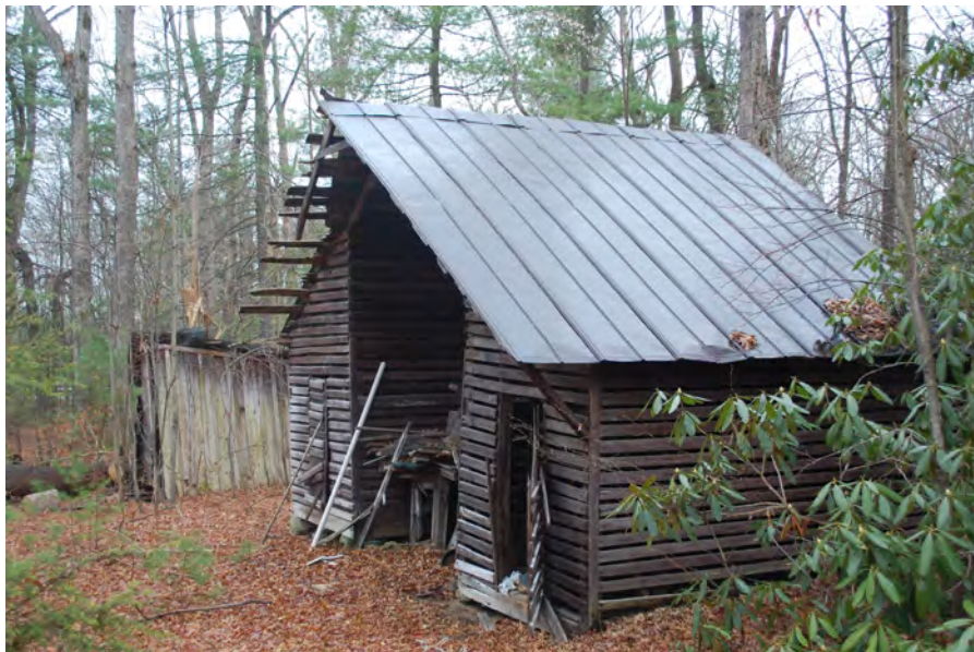
Figure 101: Crib, facing northwest
