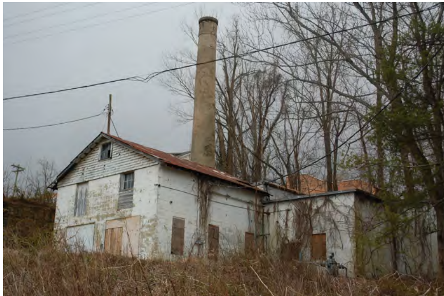
Figure 78: Boiler house, facing northwest
