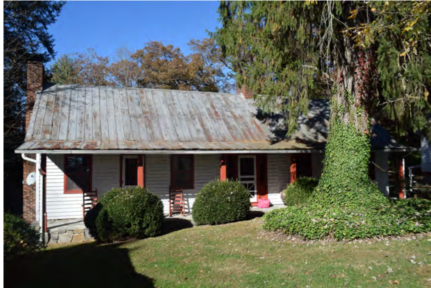
Figure 7: The Shanty, facing northeast
