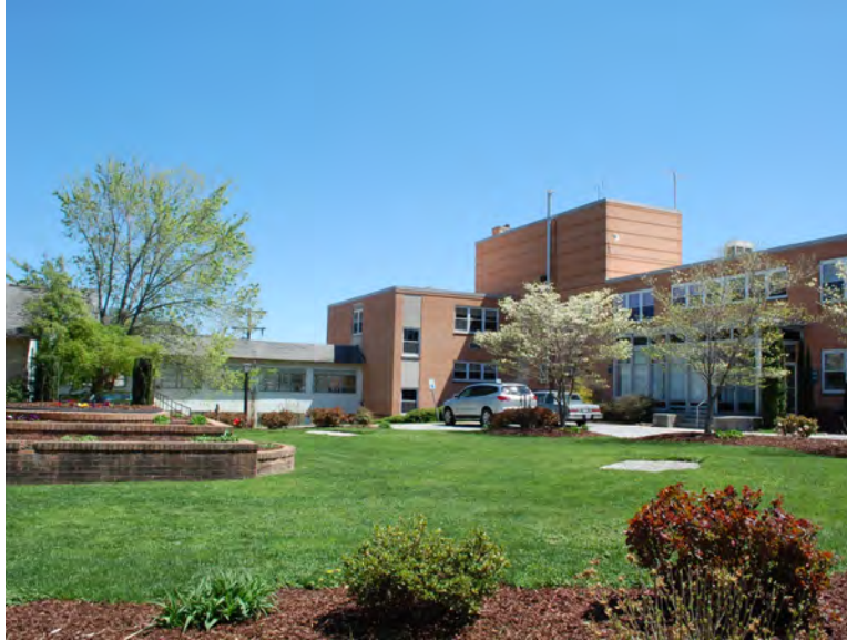
Figure 75: Circa 1950 hospital, facing southeast
