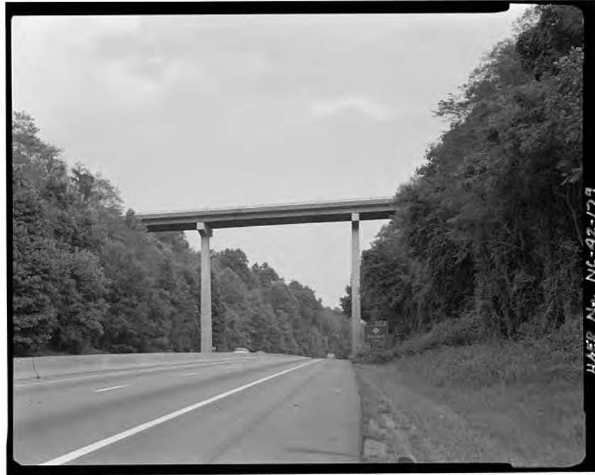
Figure 29: Bridge from Interstate 26 in 1992, facing south, from the Library of Congress
