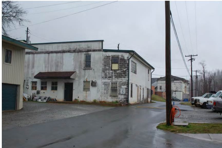
Figure 86: Rear of Maintenance Building, facing north
