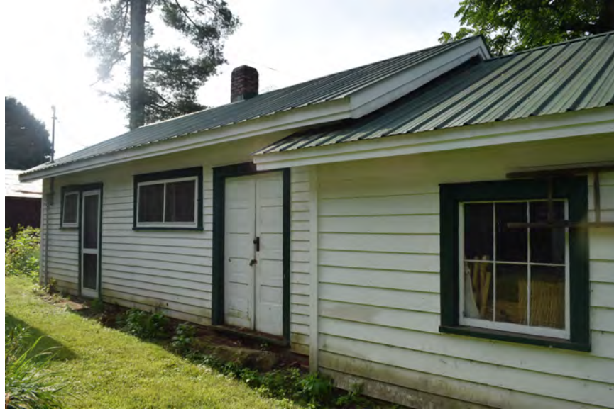
Figure 47: Wash house and garage, facing southeast
