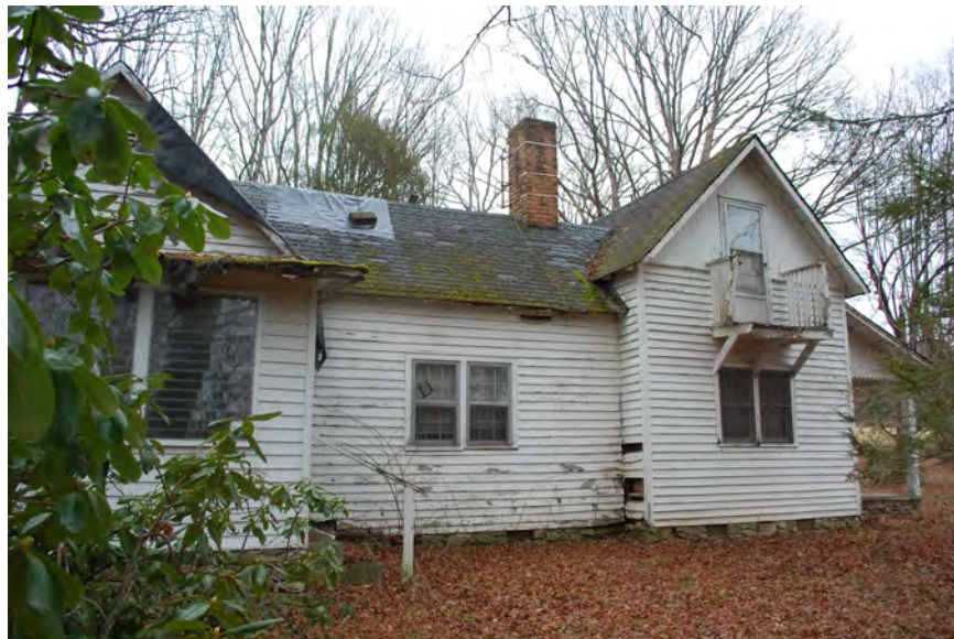
Figure 100: Justus House west elevation, facing east-southeast
