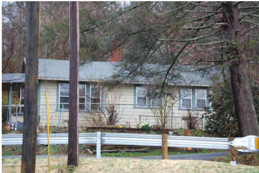
Figure 92: Circa 1930 on the west side of Howard Gap Road, facing west
