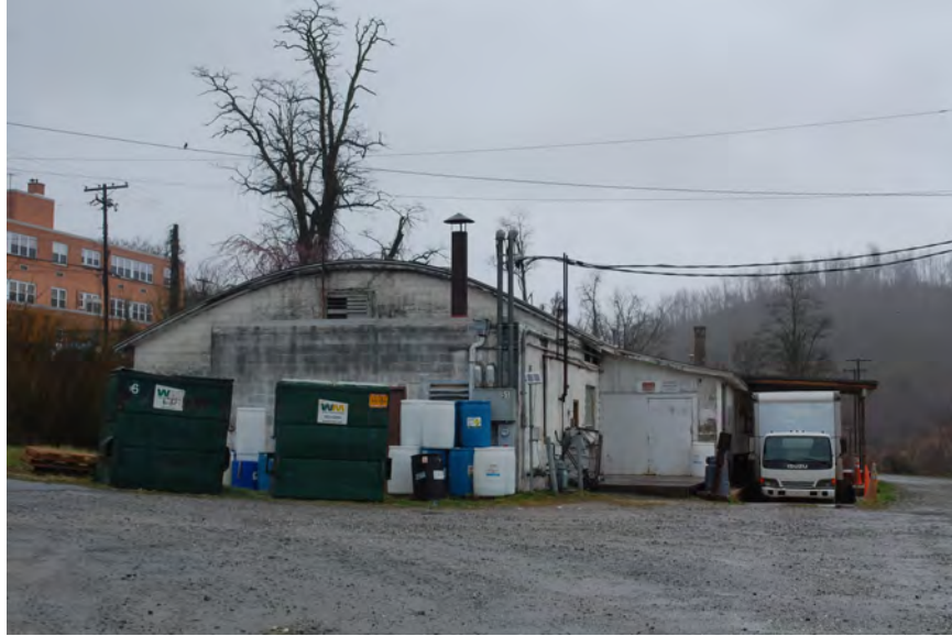
Figure 87: Circa 1950 laundry building, facing northwest
