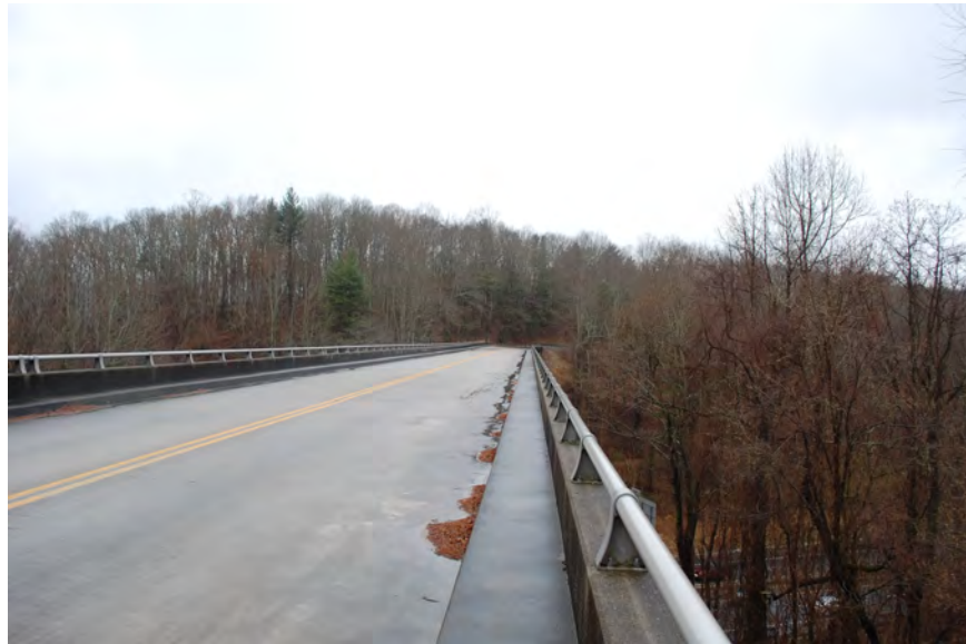
Figure 32: Blue Ridge Parkway Bridge, facing west
